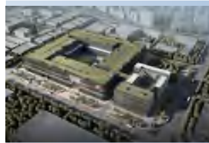
Starting construction of Han's Laser Global Manufacturing hub
